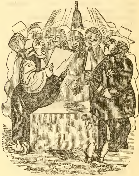
Laying the First Stone of an Hospital
